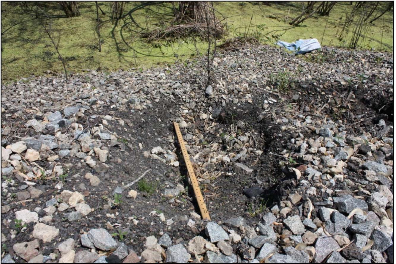
**One of approximately 26 sinkholes near the EJ& E tracks (note green standing marshy waters at the top of the photo.) The sinkholes span a distance of approximately 300 feet. CN has filled them in with gravel at least five times since the spring of 2010.**
